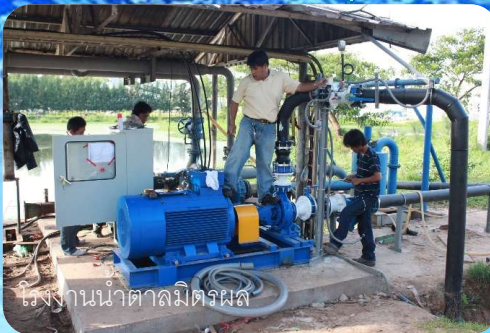
Sprinkler Pump 180 hp
