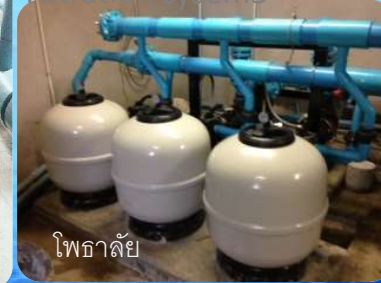
Swimming pool Filtration system 5"
