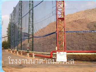
Install Pipe Steel
