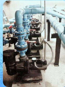
Swimming pool Filtration system 5"
